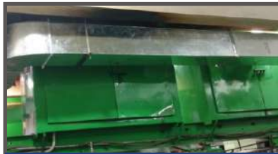
Exhaust Ducting Work
