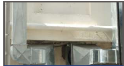
Exhaust Ducting Work
