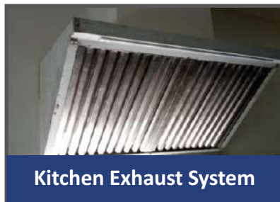
Gi Exhaust Hood With Baffle Filters
